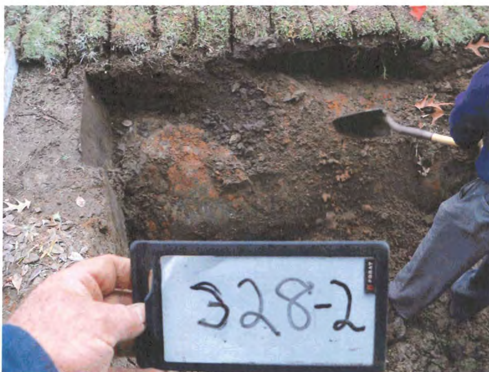
Picture 4: Excavation of UST 328-2.
